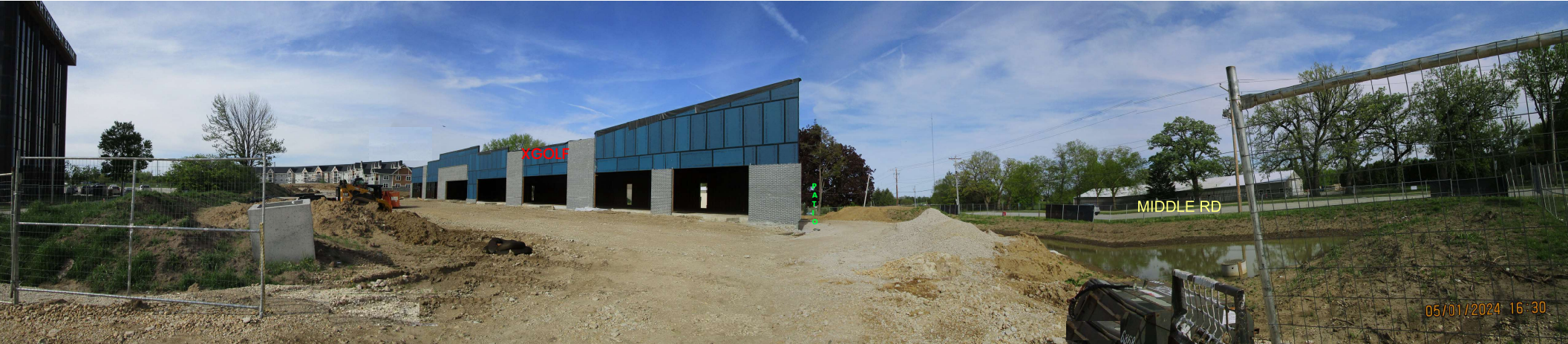
VIEW LOOKING FROM SOUTHWEST ENTRY
